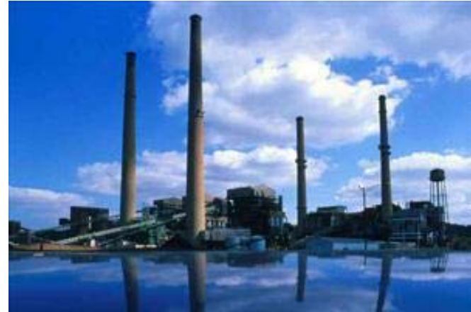
Conesville Power Plant, Coshocton, OH
